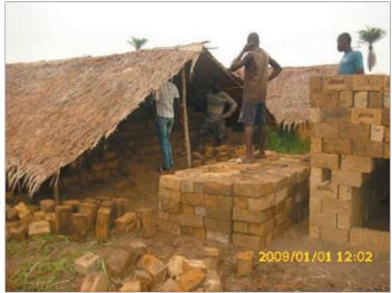
Dried bricks are mounted into a kiln. Then they are covered with mud and burned, to test their quality.
