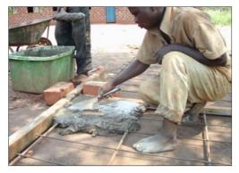
Water reservoir constructed (I), cement ceiling formed (r) and finished (below)
